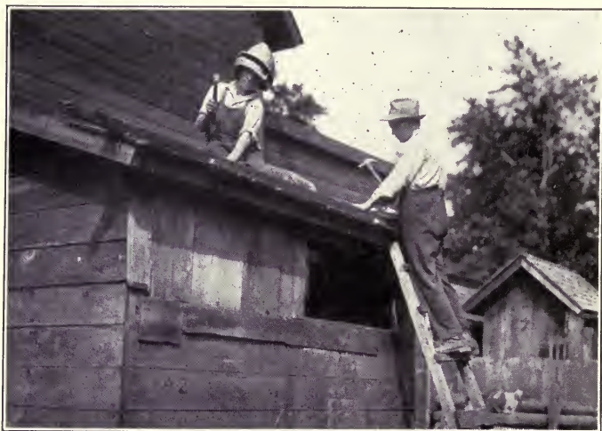
Shingling a roof. Ordinary practical work which is accompanied by a valuable trying-out process
